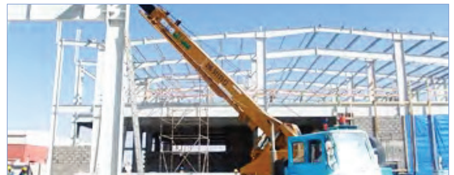
Construction at the Site
