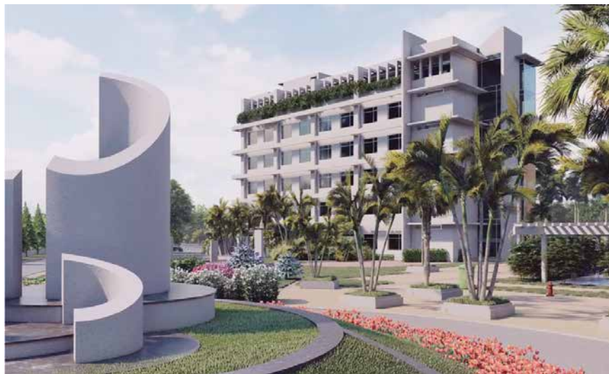
Durgapur office campus (HQ)
